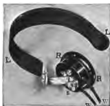
FIG. 50.—Head Telephone.
